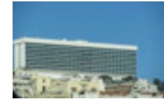
El Aurassi Hotel Renovation
